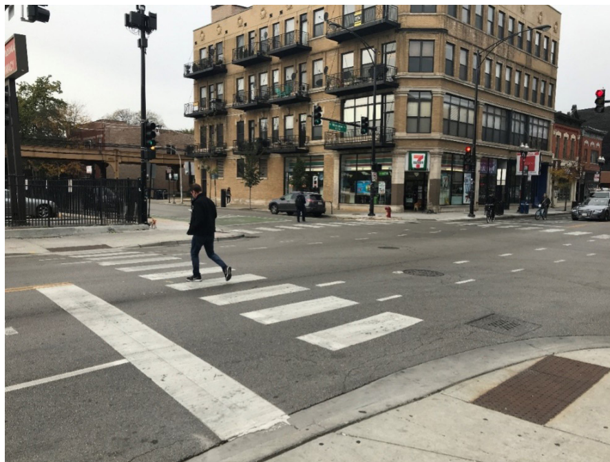
Figure 13. High-visibility crosswalk and advanced stop bar at a Signalized intersection in Chicago, IL.
