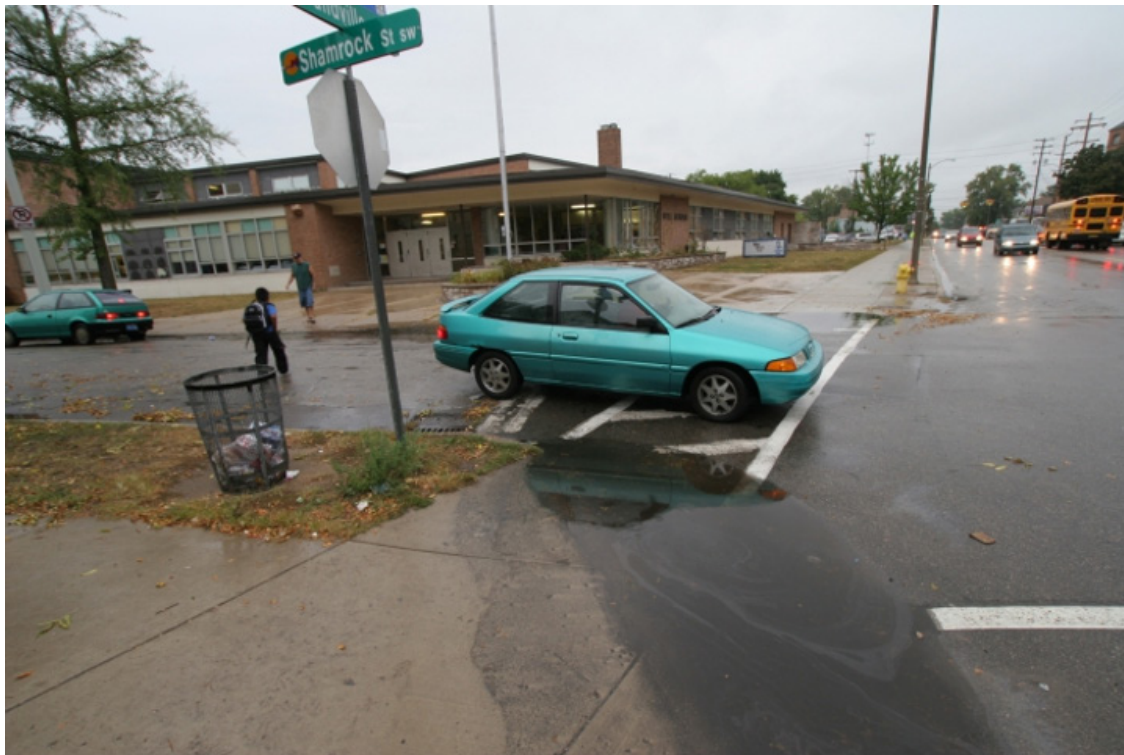
Figure 2. Example of inadequate and poorly maintained drainage blocking crosswalk. Source: Dan Burden/PBIC.
