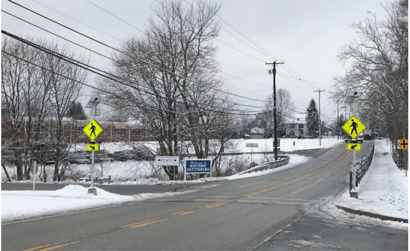
Figure 12. Example of Rectangular Rapid Flashing Beacons in Gettysburg, PA, USA.
