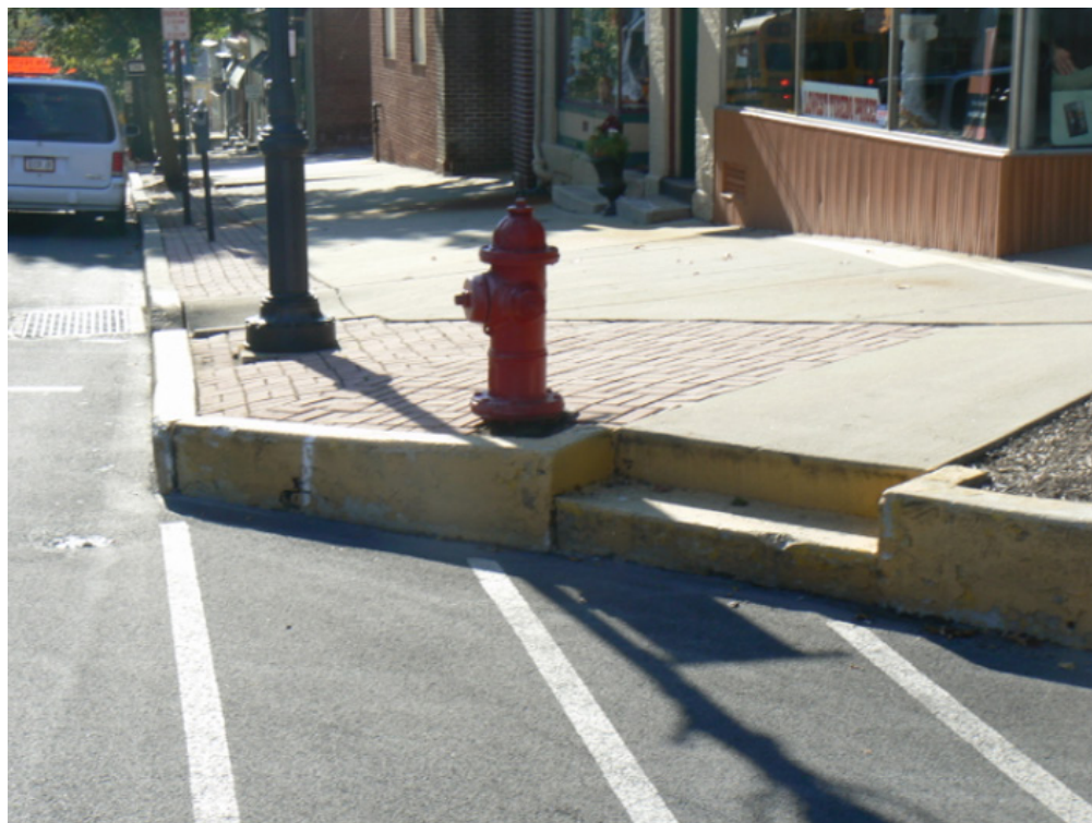
Figure 16. The ADA considers barriers to access, such as curbs and steps at pedestrian crossings, a civil rights violation and discrimination. Source: Patrick Wright, PennDOT LTAP.
