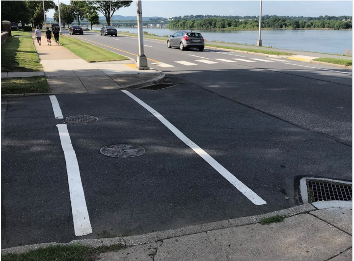
Figure 7. An example of a basic crosswalk marking across a stop-controlled approach, and a high-visibility crossing across an uncontrolled approach in Harrisburg, PA. Source: Patrick Wright, PennDOT LTAP.
