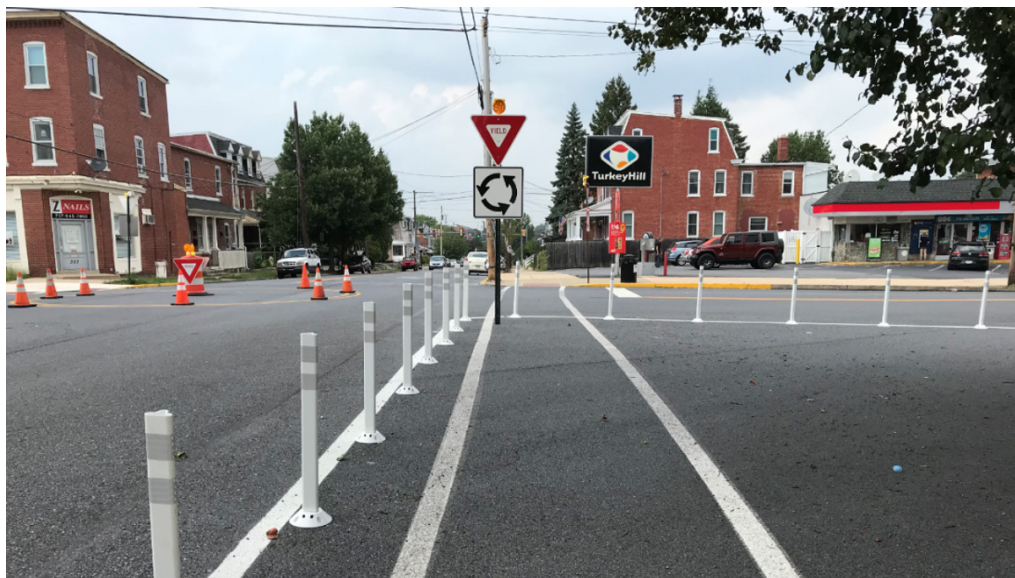
Figure 18. Temporary roundabout and curb extensions in Lancaster, PA.
