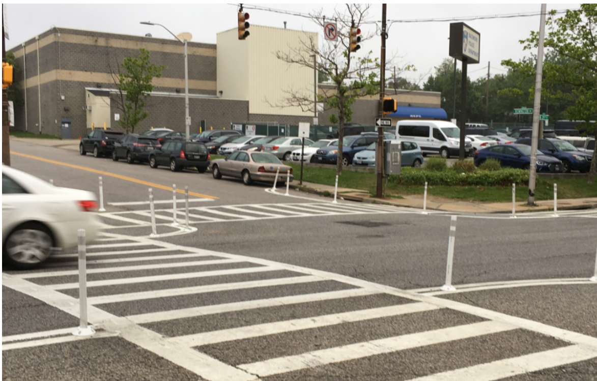
Figure 17. Example of low-cost curb extensions from Baltimore, Maryland.
