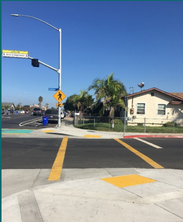
Figure 8. Image of yellow crosswalk markings in school zones required by California Vehicle Code in Imperial, CA Source: Fehr & Peers.
