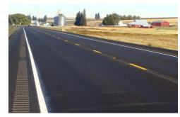
Shoulder rumble strips and center line rumble stripes are installed on this roadway.
