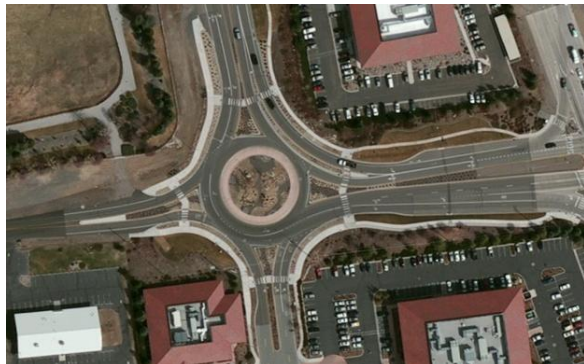
Figure 3 – Roundabout at Kietzke Lane and Neil Road
