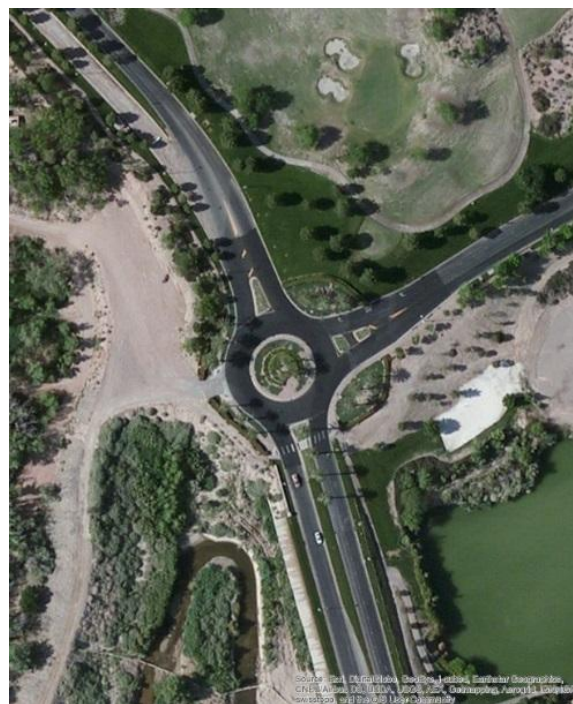
Figure 1 – Roundabout at Lake Las Vegas Parkway and Montelago Boulevard
