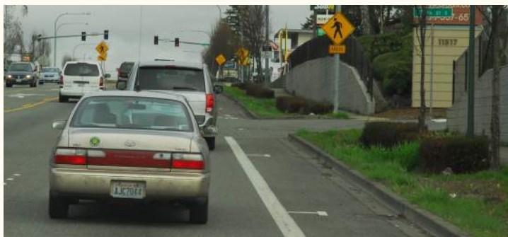
Near the intersection of SR 7 and 116th Street, there are several intersections and driveways with limited sight distance due to the retaining walls and change in elevation. The limited sight distance increases the risk in this location, where there are numerous conflict points as drivers turning left from side streets or driveways cross sidewalks, bike lanes, four travel lanes, and a two-way left-turn lane. (Credit: Dan Nabors)
