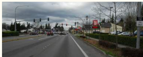
A section of SR 7 near 43rd street. The wide outside lane may encourage higher speeds. Traffic parked on the curb limits sight distance between the road and intersecting streets and driveways. Investigate the reason vehicles are parking on the curb. (Credit: Dan Nabors)
