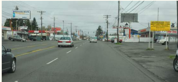
There are portions of the corridor with wide-open accesses. Wide accesses, like the one shown above, increase the potential for conflict. Creating discrete access points would reduce the number of conflict points and would increase drivers' expectancy. (Credit: Dan Nabors)
