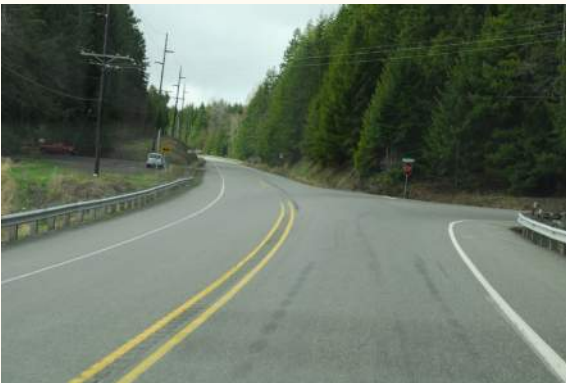
Top photo: Northbound on SR 7, near two private driveways, and heading towards the intersection with Alder Cutoff Road. Bottom photo: View of northbound on SR 7 at the intersection with Alder Cutoff Road and showing the parking area to the left. (Credit: Dan Nabors)
