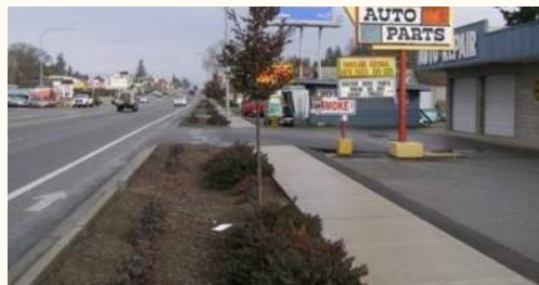
Photo top: SR 7 before implementation of access management. Photo below: the same location on SR 7 after access management implementation (Source: Analysis of Access Management Implementation: A Success Story, WSDOT). The access management project helped provide consistency in roadway cross section by defining the lanes with additional pavement markings and curb.
