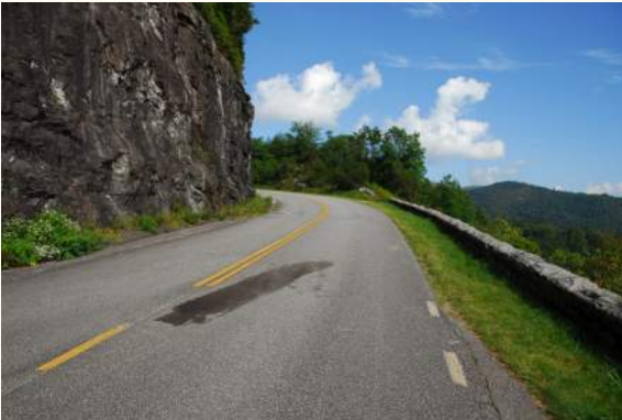
A fluid spill near mile marker 418. Fluid spills can contribute to loss of control crashes for motorcycles. This is particularly critical at this location due to horizontal curvature and limited sight distance. (Credit: Dan Nabors)
