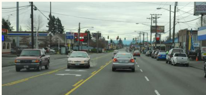
A section of SR 7 near 84th Street. There are multiple points of conflict in this section of the corridor, including left-turning vehicles from the two-way left-turn lane, traffic in the unmarked parking lanes, and vehicles entering from side streets and driveways. (Credit: Dan Nabors)
