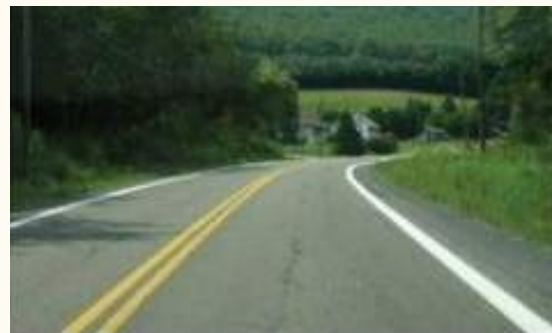
4-inch edge and center lines (top). Wider 8-inch edge and center lines (bottom). (Credit: FHWA)
